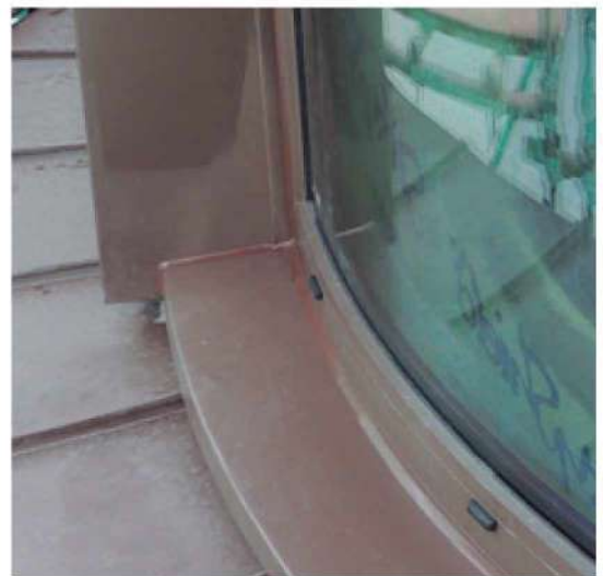
Aluminium window frame sealed against the elZinc Rainbow® Brown sill using brown neutral curing silicone
