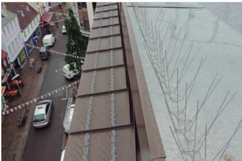
Bird spikes attached using neutral curing silicone
