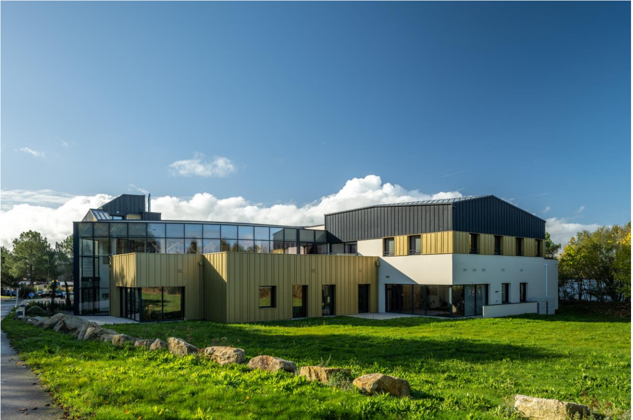
The main façade of the Sequoia Centre clad in elZinc Rainbow® Gold and elZinc Graphite® zinc.
