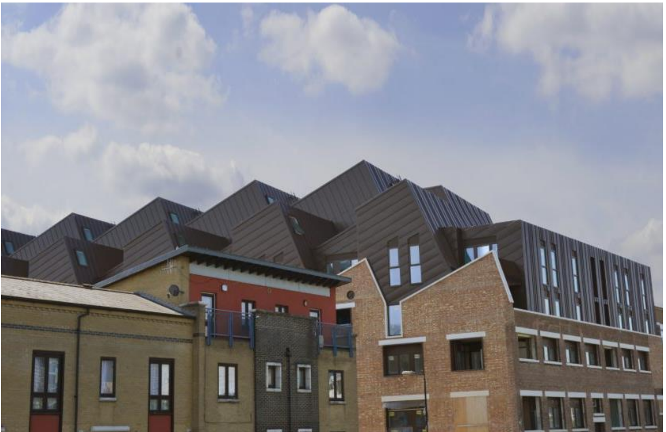
The roofing and cladding echoes the saw-tooth profile of the former factory
