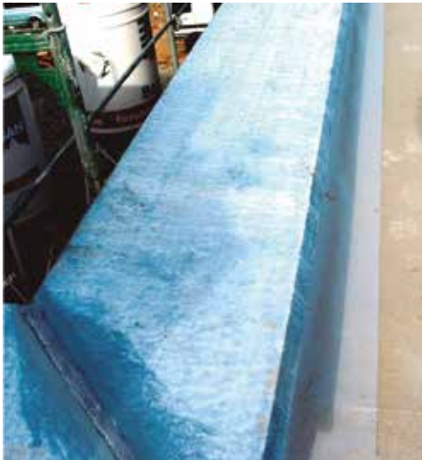
Staining caused by cement and plaster dust is costly to remove if it has stained the surface after light rain, fog or dew.
