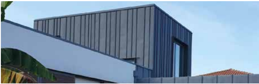
Housing development. Standing seam in zinc.
