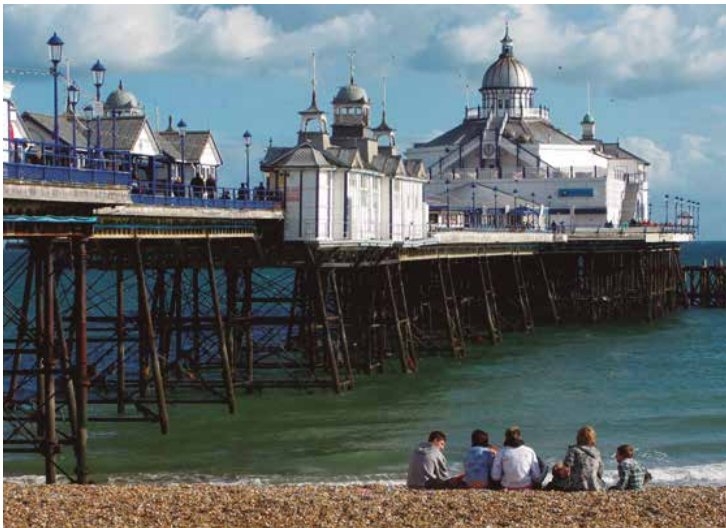
Old zinc roofs on Eastbourne Pier, England.
