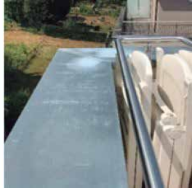
A more severe case due to ponding. Cases like this should be removed as soon as possible after they are detected.
