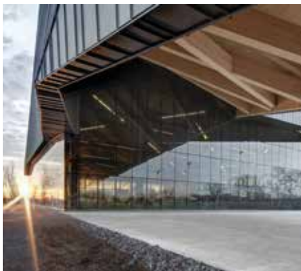
elZinc Slate®, football stadium, Montreal, Canada
