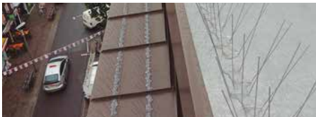
Bird spikes attached using neutral curing silicone
