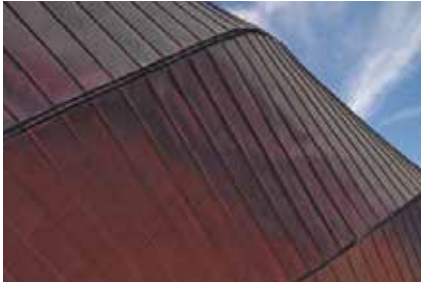
Double lock standing seam in copper
