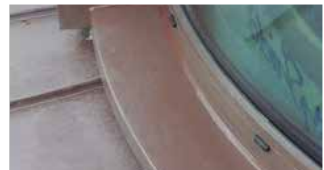
Aluminium window frame sealed against the elZinc Rainbow Brown sill using brown neutral curing silicone
