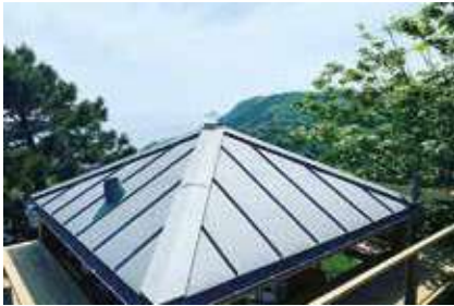
elZinc Slate® on UK Coast Housing development, England.
