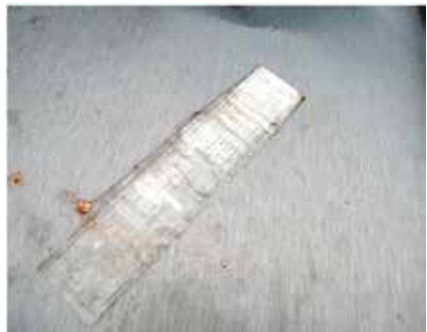
Adhesive strips should be removed from the zinc Surface as soon as detected, and any adhesive residue cleaned.
