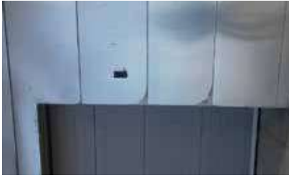
Partial removal of protective film causing differential weathering on natural zinc. These differences will weather-out over time
