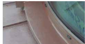
Aluminium window frame sealed against the eZinc Rainbow Brown sill using brown neutral curing silicone
