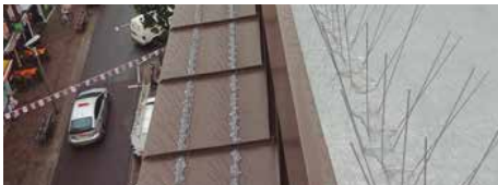
Bird spikes attached using neutral curing silicone
