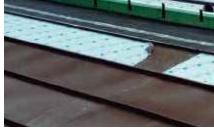
Partial removal of protective film causing marking of Rainbow brown – this can be wiped away.
