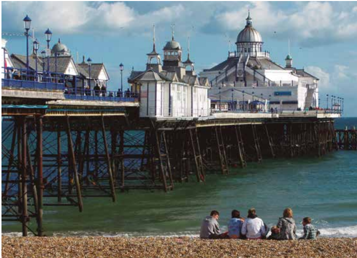
Old zinc roofs on Eastbourne Pier, England.
