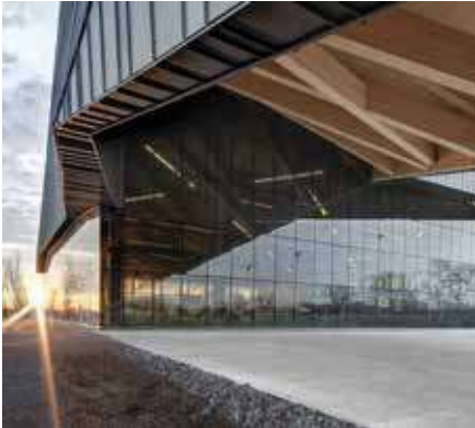
eZinc Slate®, football stadium, Montreal, Canada
