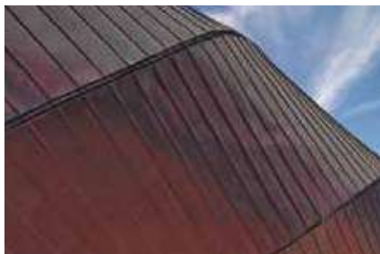
Double lock standing seam in copper
