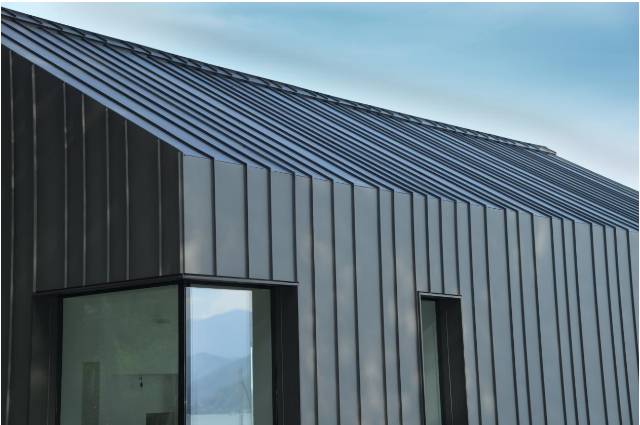
The deck and façade have been completely clad in zinc.
