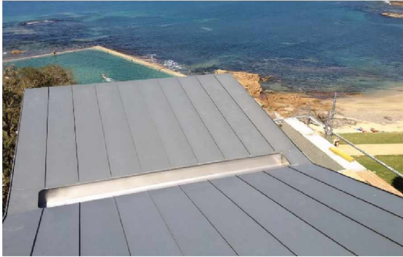
Frequently rain-washed areas do not allow salt deposits to build – eZinc Slate at Fairlight, Sydney
