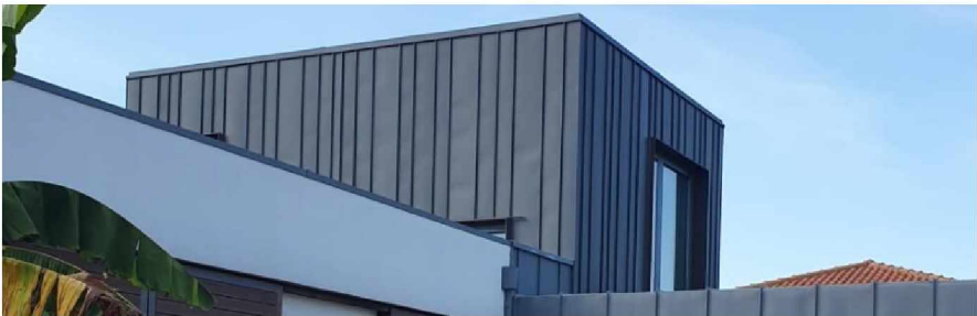
Housing development. Standing seam in zinc.
