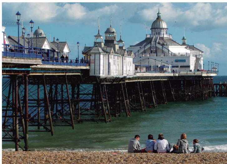
Old zinc roofs on Eastbourne Pier, England.
