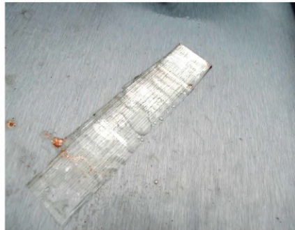
Adhesive strips should be removed from the zinc surface as soon as detected, and any adhesive residue cleaned.
