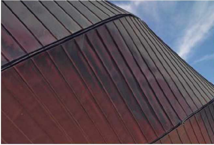
Double lock standing seam in copper
