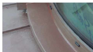
Aluminium window frame sealed against the eZinc Rainbow Brown sill using brown neutral curing silicone
