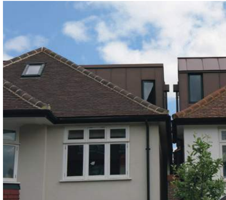
Roof extension, Wimbledon, London, UK Ultra Violet Designers, Architects Ltd.
