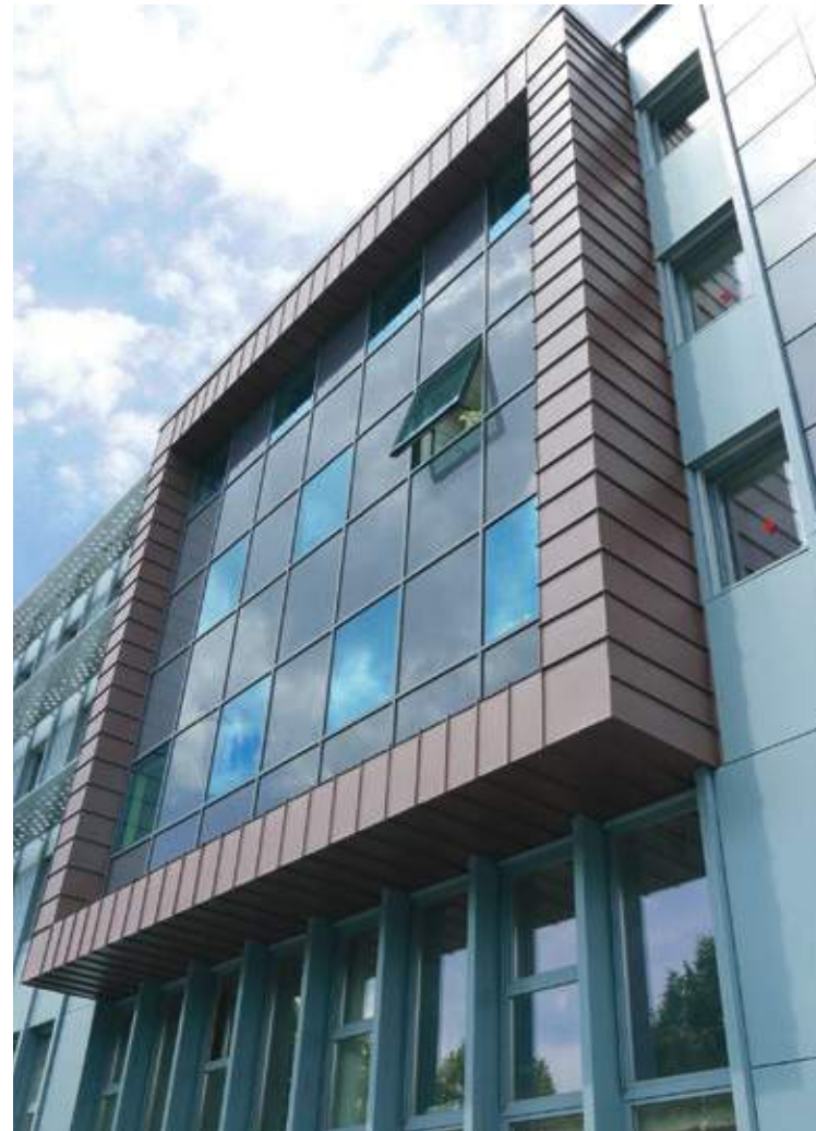
Office building, France - Jean-Paul Faure.
