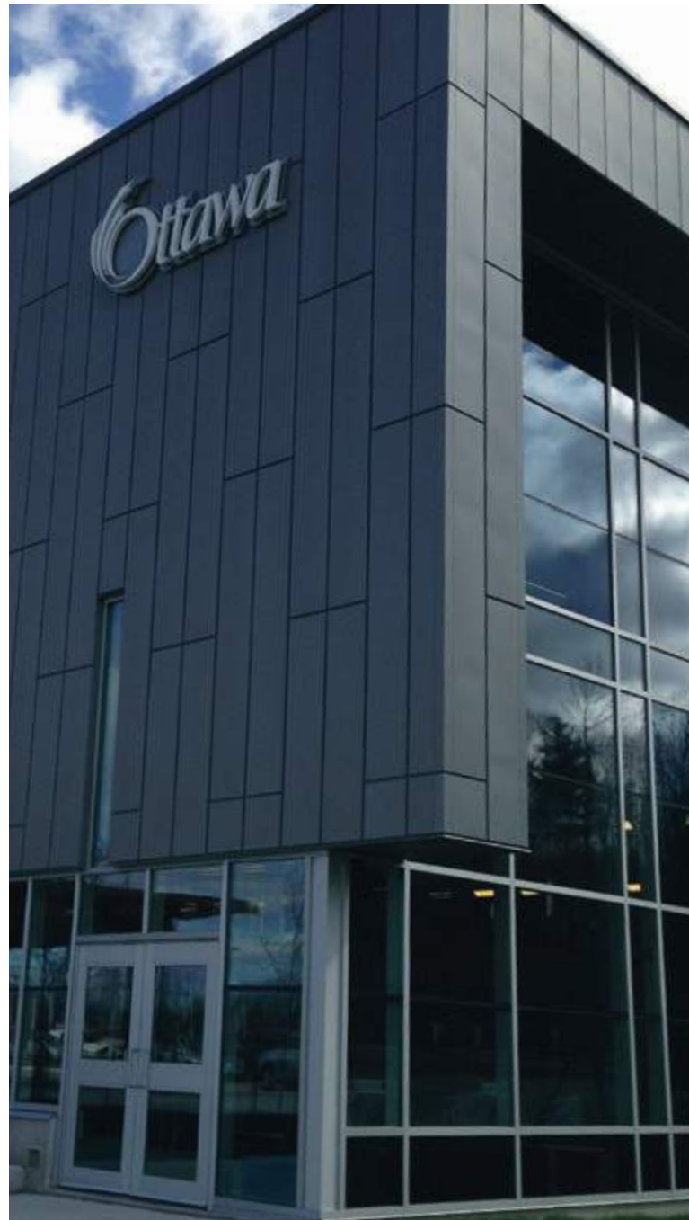
Richcraft Recreation Complex, Kanata, Ontario, Canada Salter Pilon Architecture Inc.
