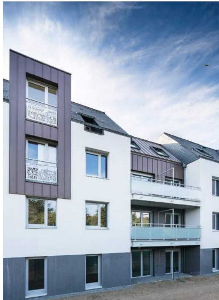
Residential development, Pornichet, France - ASA Gimbert.
