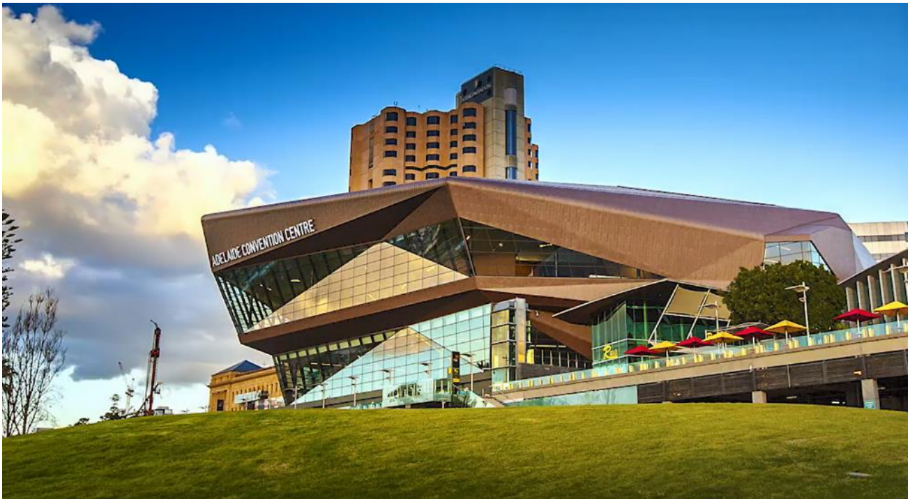
The external shape of the building and the red coloured zinc cladding were inspired by the granite rock formations known as The Remarkables.
