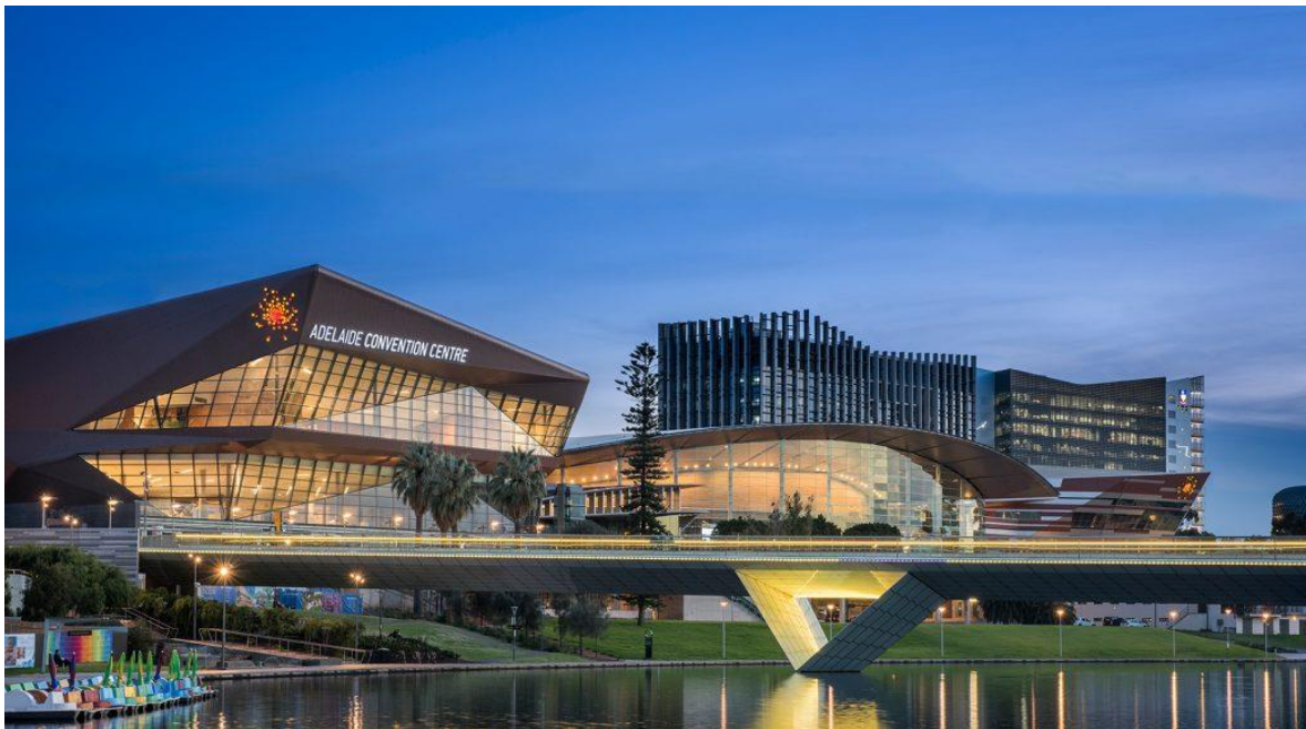
Zinc Ibérico and elZinc Rainbow red were chosen to clad the Adelaide Convention Centre in Australia Architect: Woods Bagot Adelaide
