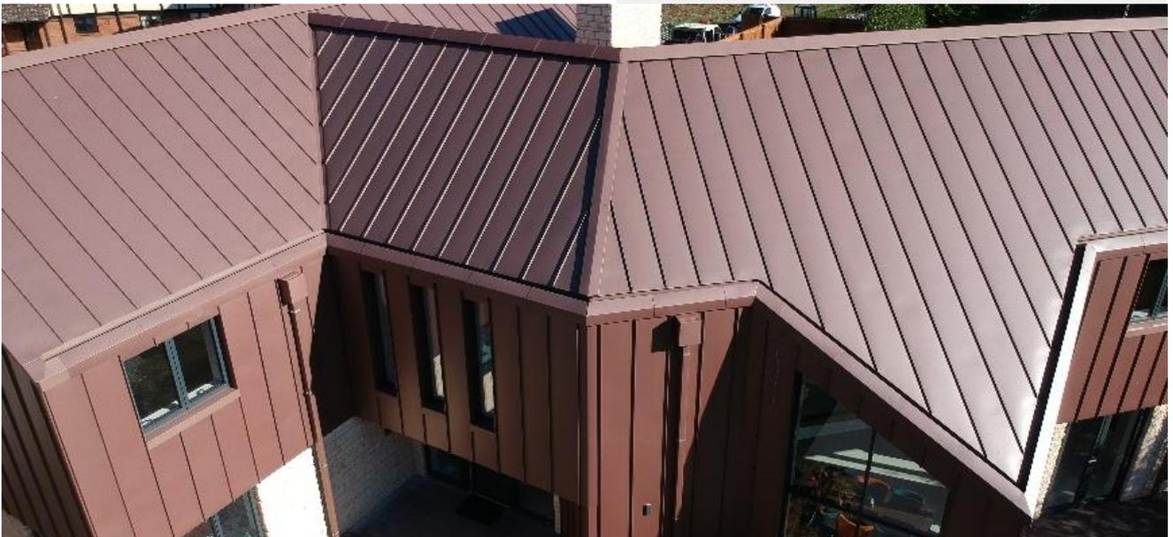
*The gutters in the eaves recede and hide inside the deck.*
