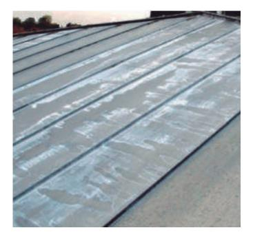
The effect of deficient protection allowing moisture in between windings on a coil prior to installation. The same effect is possible wherever water is trapped for long periods, and even if the stains do not immediately appear after installation, the route cause is clear.
