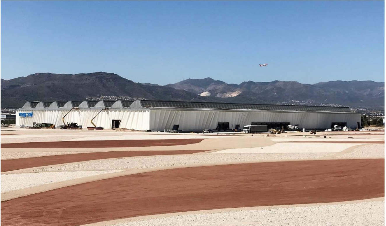
The materiality of zinc as a roof cladding fits in perfectly with the original design of the factory. Pictures : courtesy of Rafael Urquiza Sánchez
